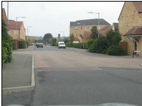
Speed Table on Woodcock Rd and Siskin Close with lack of road markings
