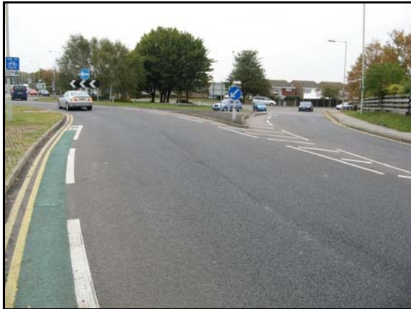
Old North Rd South approach with cycle lane to be extended and traffic lane to be widened to 2 lanes
